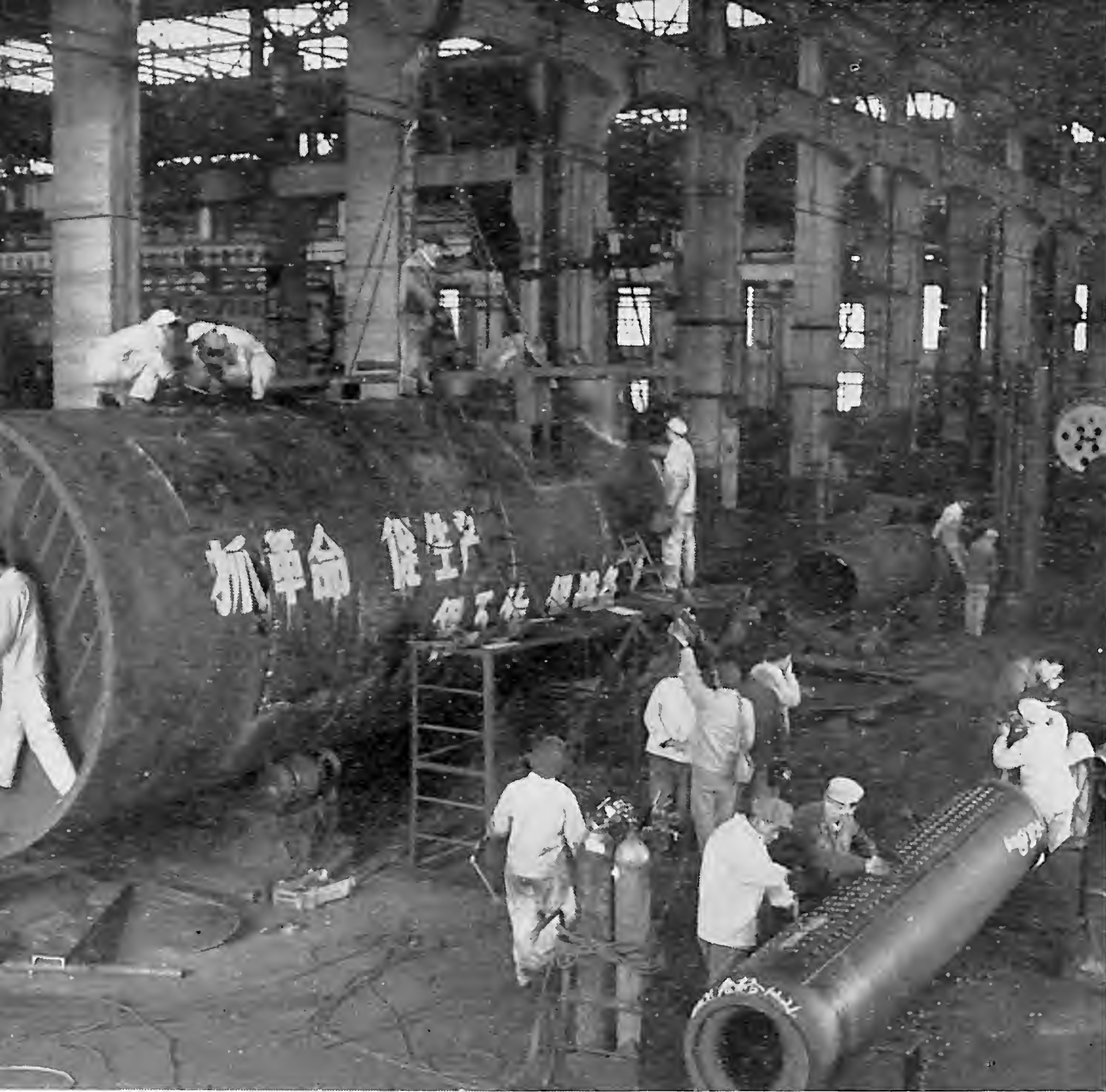
A shop in the boiler plant.
